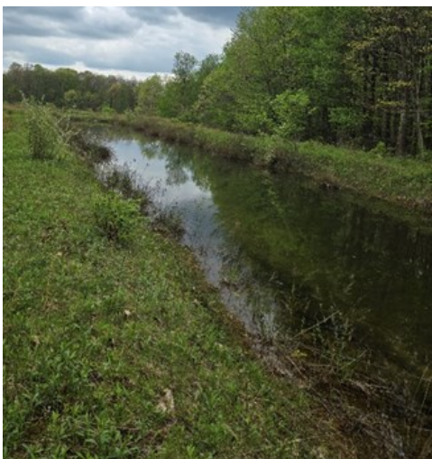
Forebay at De Sale Phase II
