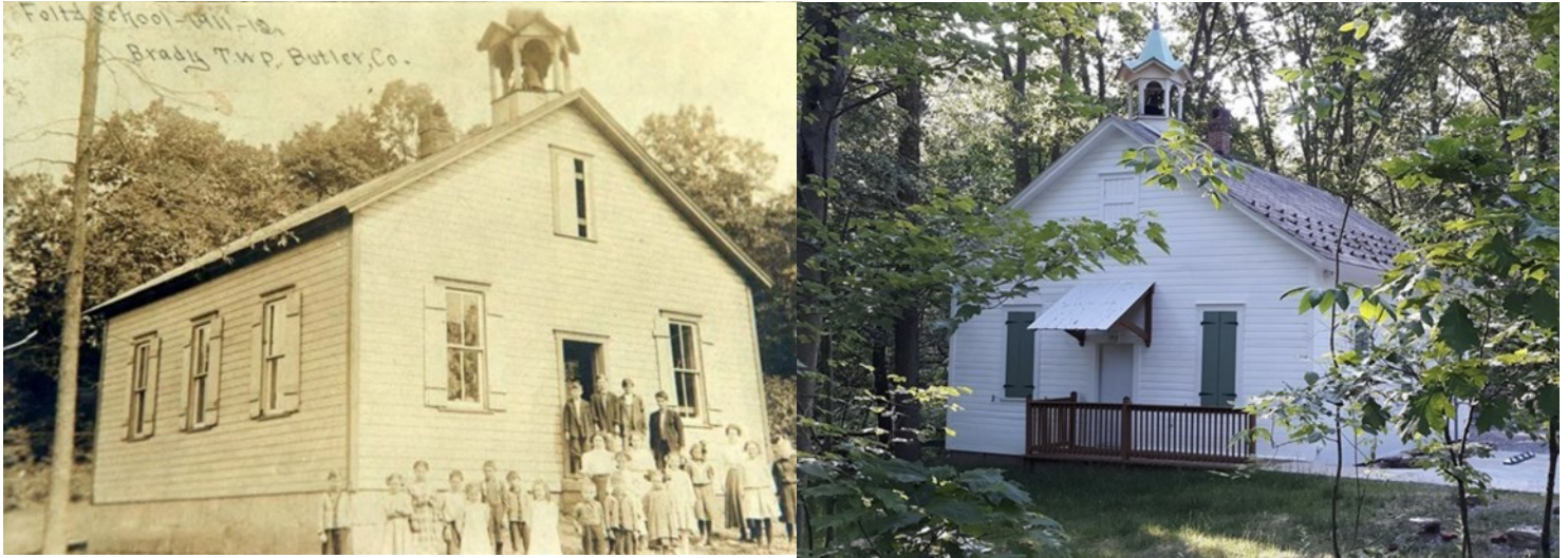
Photo of Foltz Schoolhouse in 1900's (Left) versus today following renovation (Right).
