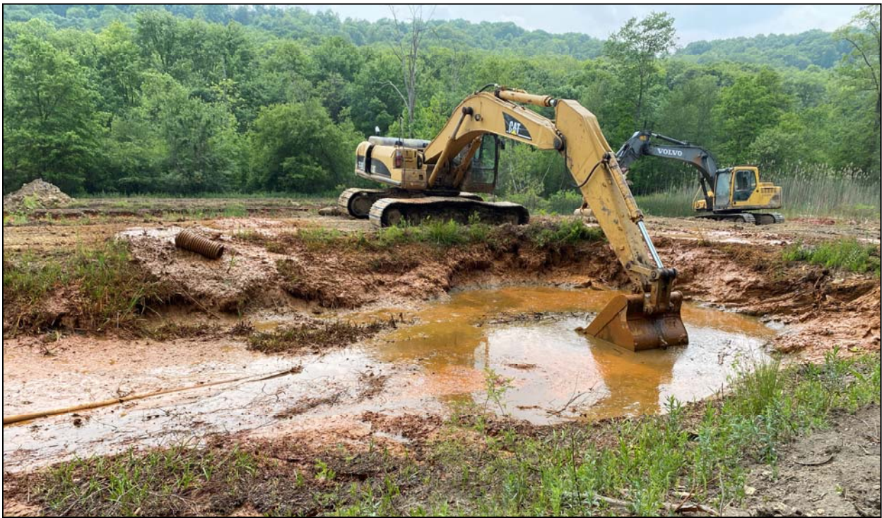
Spur Excavation, LLC removed all of the iron precipitate that had accumulated within the aerobic wetlands and placed in a newly constructed sludge pond.
