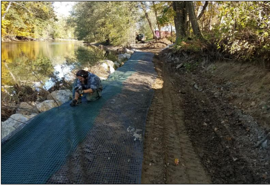
Cory Mahony installing staples within the first soil lift at the Slippery Rock Campground stream bank restoration project.
