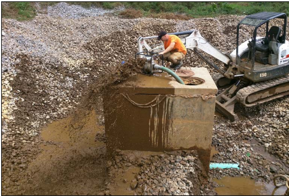
BioMost intern Cam Thon pumping sludge out of the AFVFP siphon vault at the McIntire passive system.
