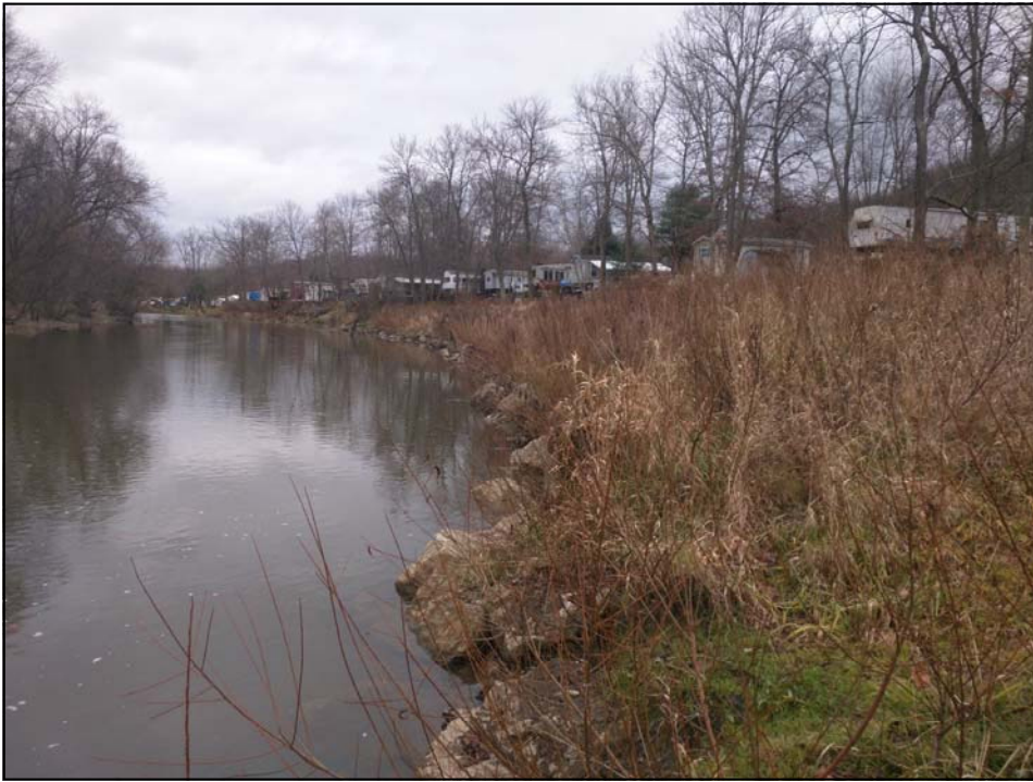
Photo taken in December 2016 of the stream bank restoration project completed in the fall of 2014 at the Slippery Rock Campground. The bank has become well vegetated with willows approximately 3' tall.
