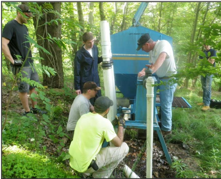
Jennings staff working with Josh Matheny , Aquafix Engineer, and BioMost, Inc. personnel to retrofit an existing Aquafix® lime-doser with a 24-volt generator system referred to as a “Trickle Charger”. See article on first page.
