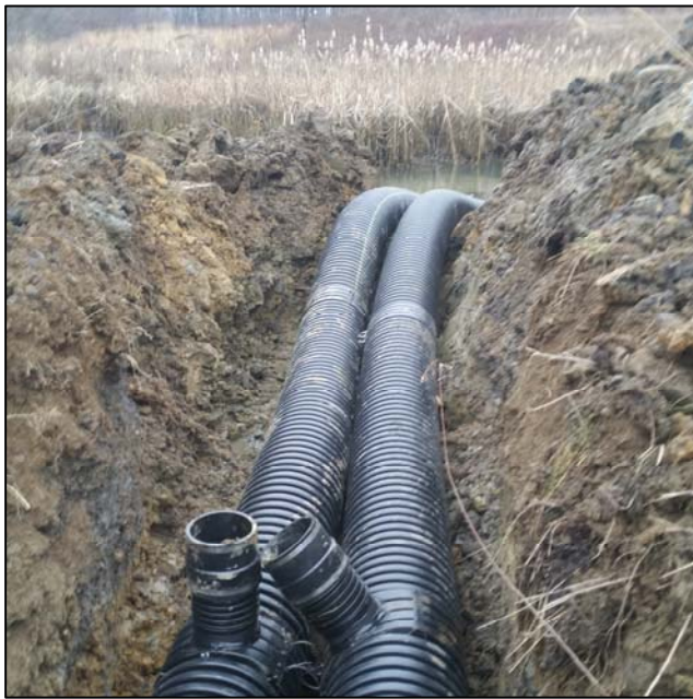
12" culvert pipes with cleanouts to reduce beaver activity at De Sale Phase II (Left). The access road to the system was flooded due to water overtopping the berm of the wetland (Right). See article on first page for more information.
