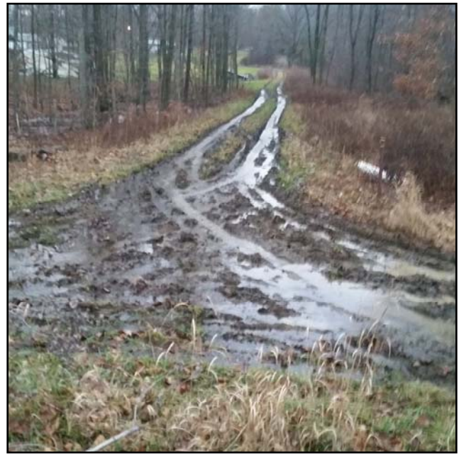
12" culvert pipes with cleanouts to reduce beaver activity at De Sale Phase II (Left). The access road to the system was flooded due to water overtopping the berm of the wetland (Right). See article on first page for more information.
