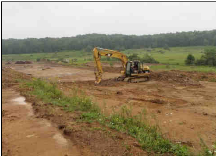
Joe Puryear excavates part of the wetland.
