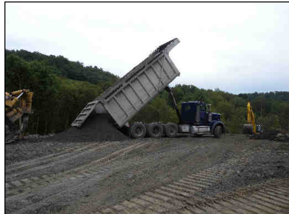
Mineral CSA is unloaded & mixed with non-commercial refuse.
