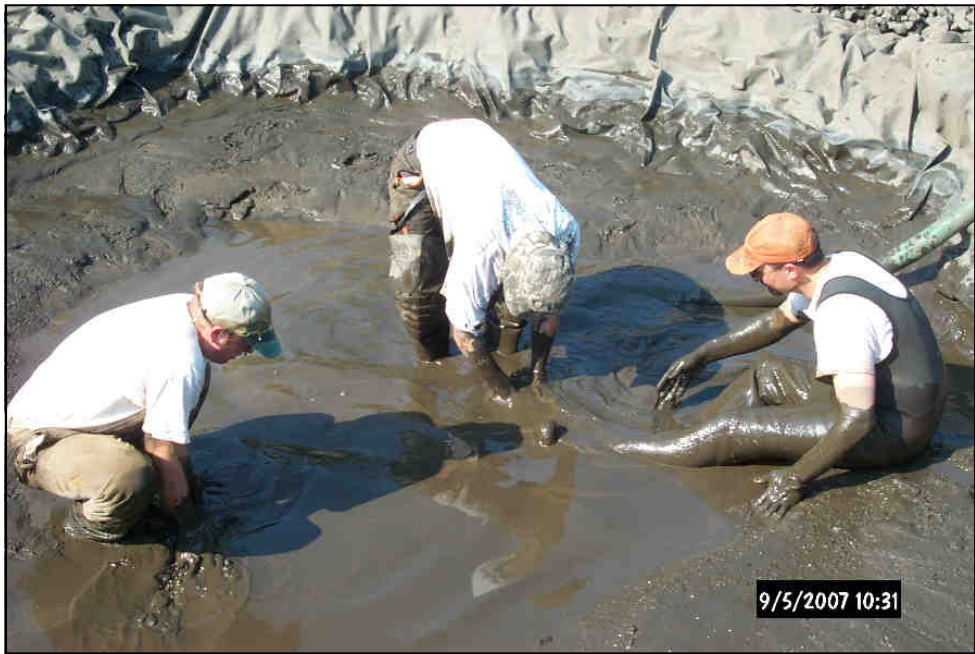
Playing in the Mud Shaun Busler, Tim Danehy, and Cliff Denholm pumping the manganese material cleaned from the limestone to a dewatering bag. (See article on page 1.)
