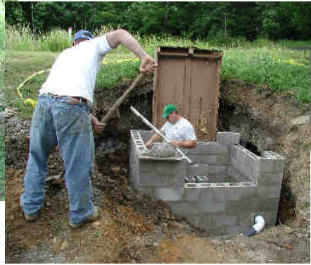
The new vertical flow system flow control box (right) at Jennings Environmental Education Center took a lot of work to construct (center), but was in need of repair (old VFS flow control box pictured at left). Please see article below.
