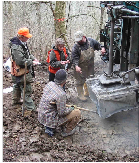
Herschel Mathews, Jr. (landowner) and Buddy Pecjak installing drill roads for Mike Hollobaugh and John Ridings of McKay & Gould Drilling to install piezometers at the Dunkard Creek AMD Project.
