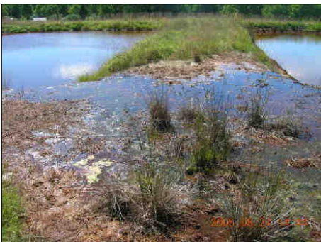
Left: The two vertical flow ponds are designed to function in parallel. However, due to iron minerals forming at low pH, the flow distribution system frequently plugged, causing unbalanced overland flow.
