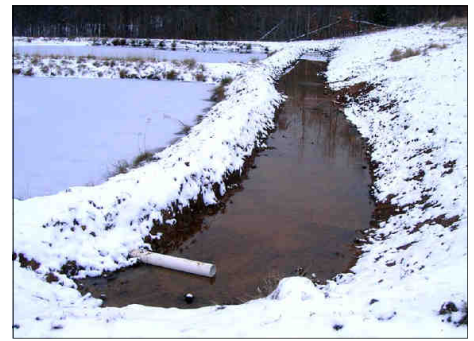
Left: The two vertical flow ponds are designed to function in parallel. However, due to iron minerals forming at low pH, the flow distribution system frequently plugged, causing unbalanced overland flow.
