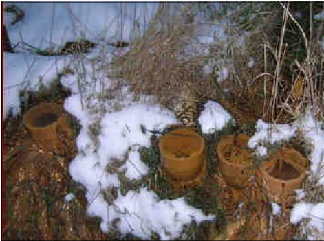
Left: The existing outlet pipes prior to removal.
