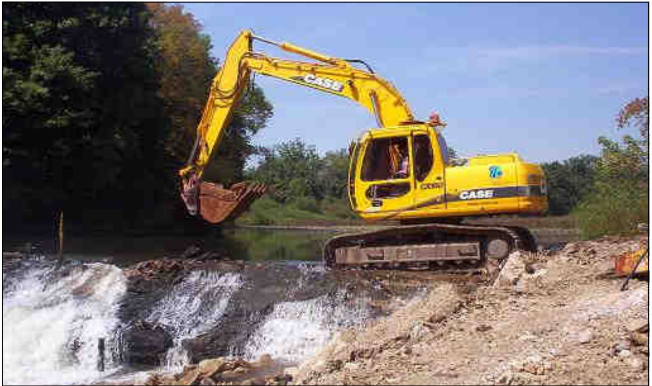
An excavator begins to breach the dam across Wolf Creek, slowly lowering the impounded water. (See article below)
