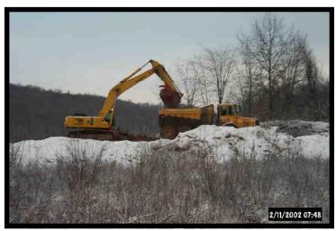
Construction activities are well underway at the Erico Bridge Restoration Area. The photo to the left shows Quality Aggregates personnel removing the acidic coal refuse (gob) from a pile located within Seaton Creek. A naturally functioning wetland specifically designed to maximize wildlife potential as well as provide water treatment will be constructed in the foot-print of the barren gob pile.
