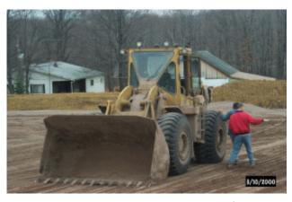
Passive treatment system with vertical flow pond under construction.
